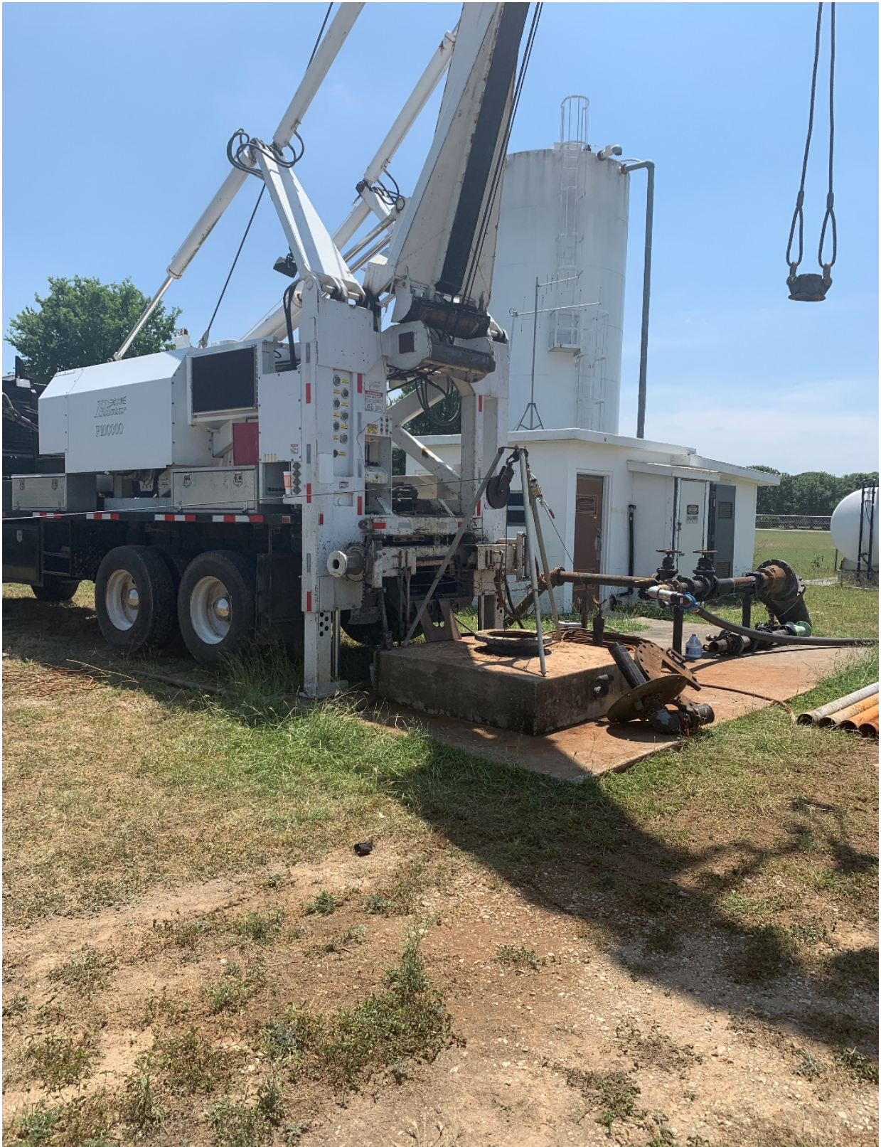
Photo (courtesy of RESPEC) of the Peerless crane truck to conduct well testing at the Medina Valley Water System Well.
